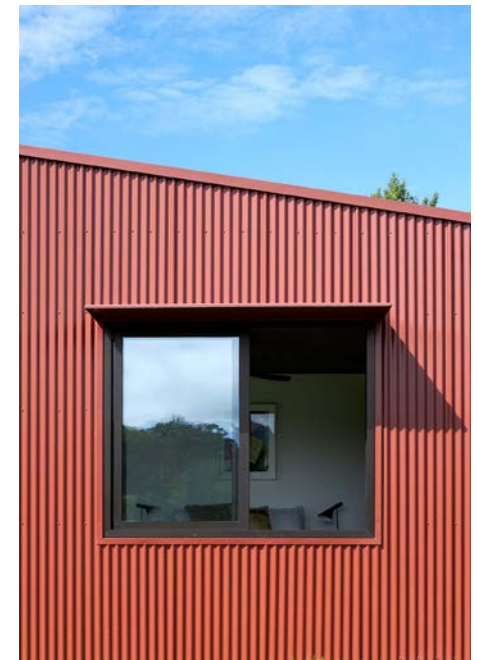
Acceptable window proportions with sun shading devices to reduce over heating
