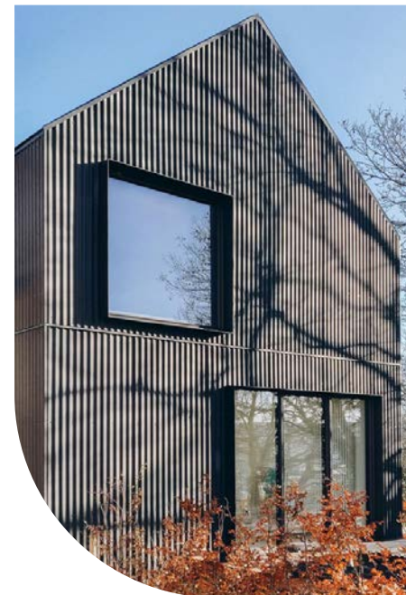
Acceptable window proportions with sun shading devices to reduce over heating
